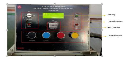
Station Master's Key (with ON/OFF or IN/OUT Position)
